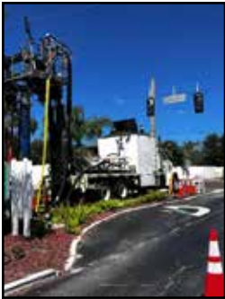
Pipe-lining equipment at 8th Avenue entrance.
